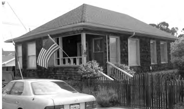
*125 15th St. Asbestos shingles have been removed to reveal the original wooden shingles*
