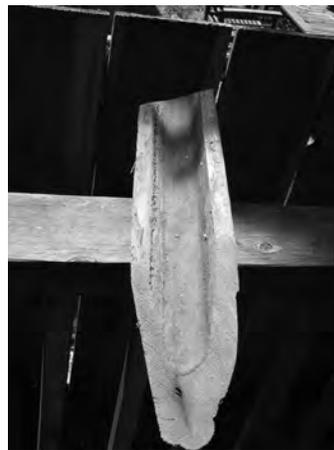
*A section of wooden gutter*
