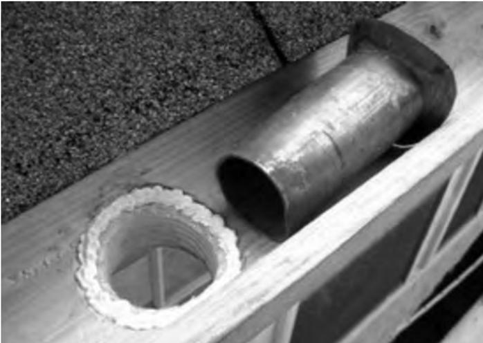
*A new wooden gutter, with a new downspout hole, and new lead downspout leader, ready to be installed.*
