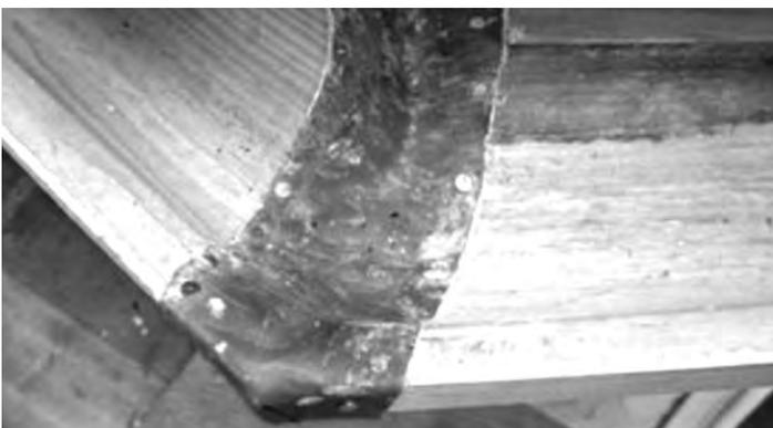
*The same inside corner with new gutter, and lead flashing installed and caulked.*
