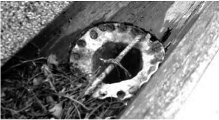
*An old wooden gutter, with an old downspout hole, and old lead downspout leader, ready to be replaced.*
