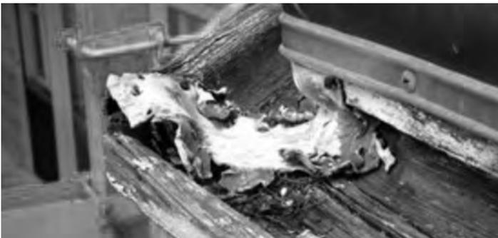
*Typical worn-out beveled intersection of 2 gutter pieces, with lead flashing.*
